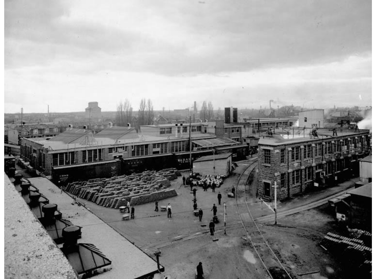
Fairbanks-Morse complex looking northwest, 1914. LAC a024502.
