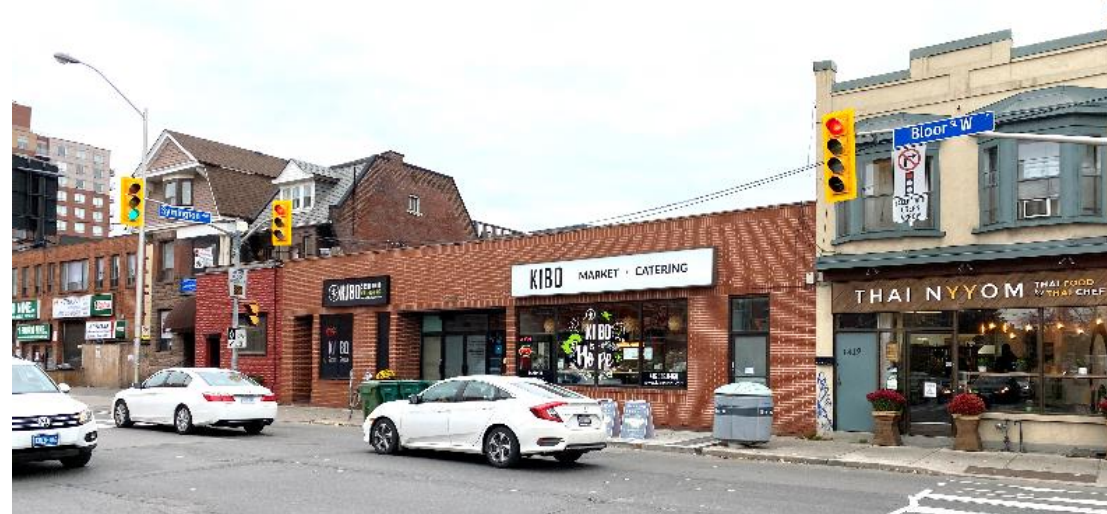
Commercial uses along Bloor St W at Syrington Ave
