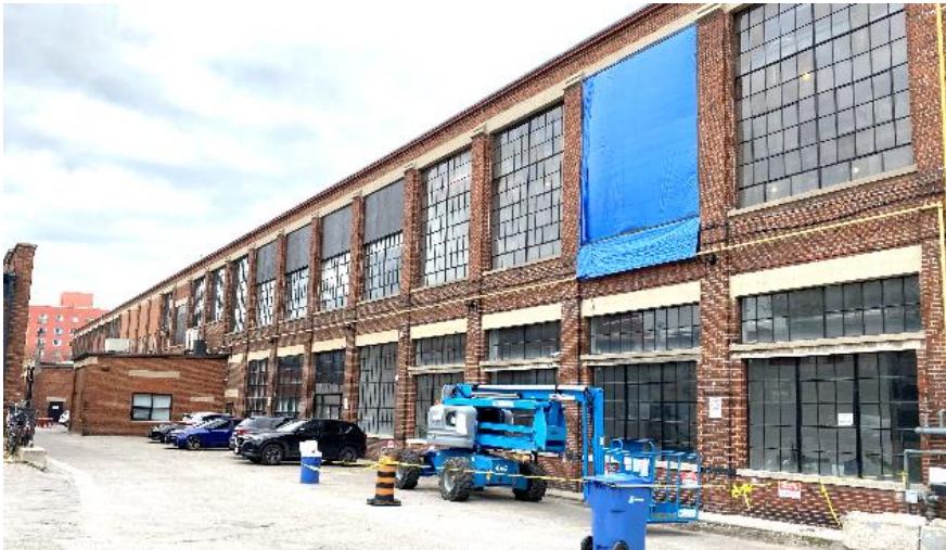
North elevation of 219 Sterling Rd
