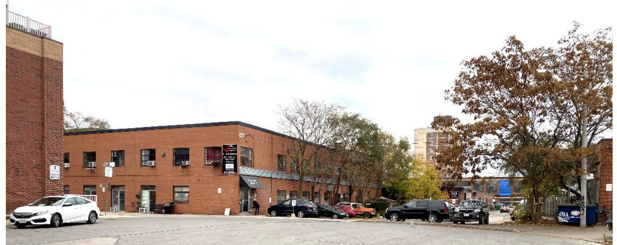
Ruttan St, looking south towards 227 Sterling Rd
