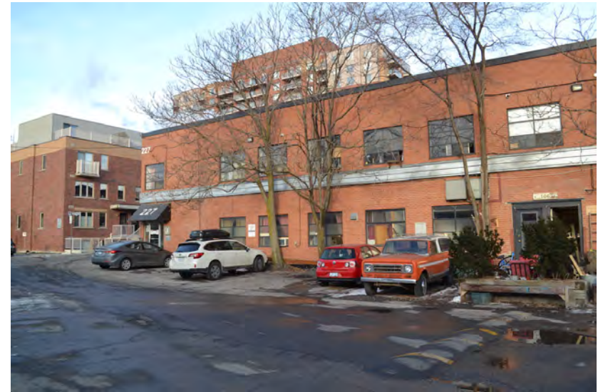
Figure 15 - View of the west facade of Building A.
