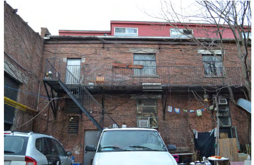
Building B (east) east elevation, showing new doorway at second level fire escape, and new red cladding and window units at clerestory window.
