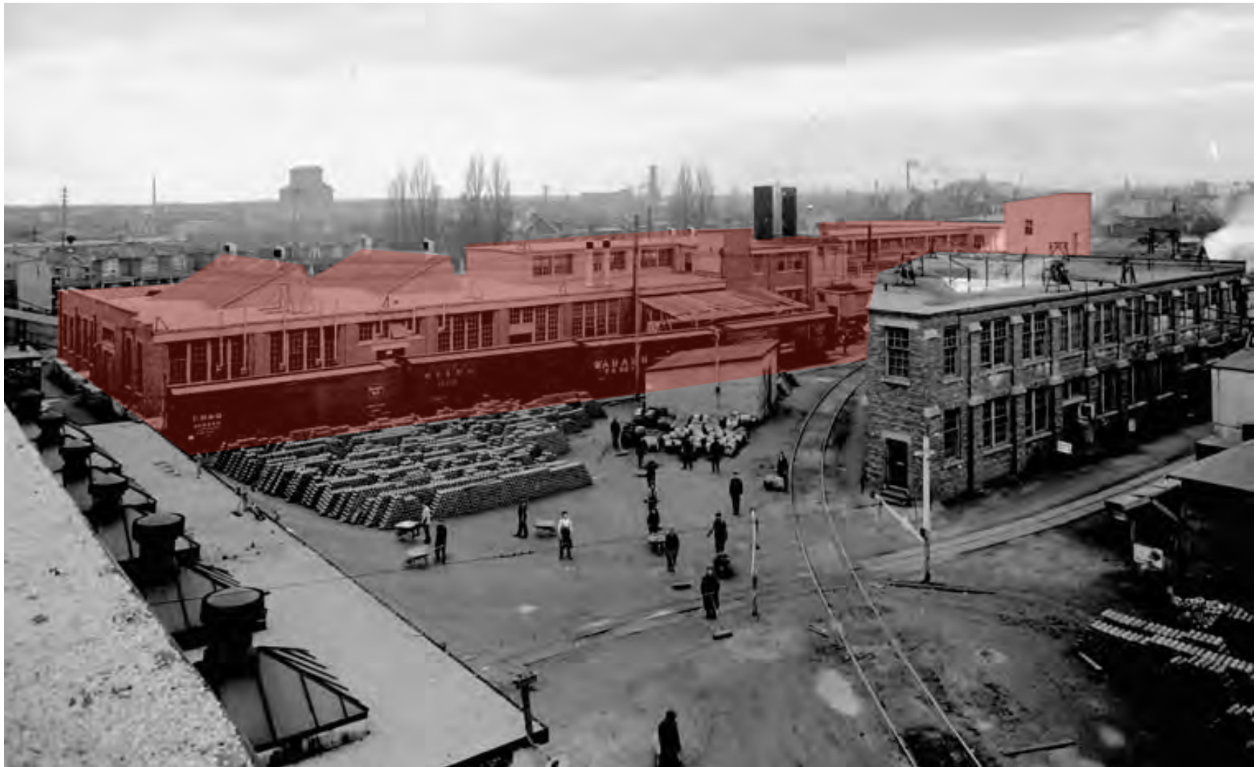
Aerial photograph of the subject site, highlighted in red, looking northwest from the roof of 213-219 Sterling Road, c1914-1918. Section of the Canadian Fairbanks-Morse Co. Ltd. manufacturing Department, Toronto, Ontario (Library & Archives Canada, a024502).
