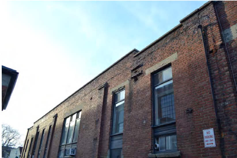
Figure 17 - View of Building C, showing a transition at pilasters between construction phases at the south elevation.
