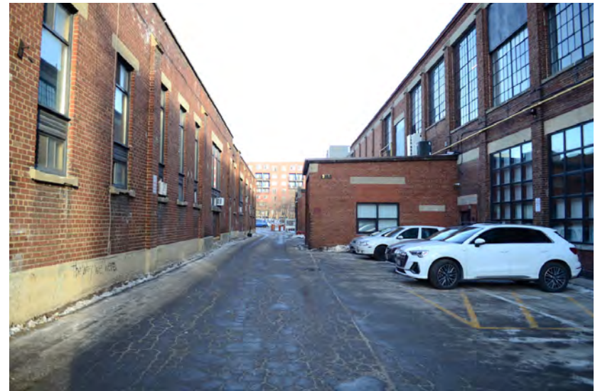
Figure 3 - View of the right-of-way, looking east, showing the subject site south facade to the left and former Moloney Electric Building.
