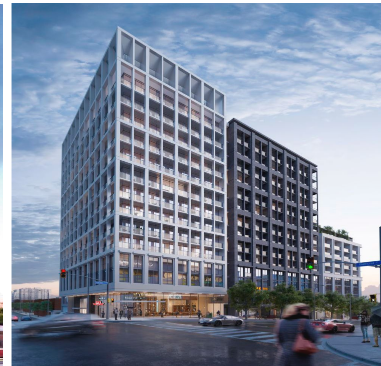
875 Eglinton Avenue West, The Forest Hill (14 Storeys)
